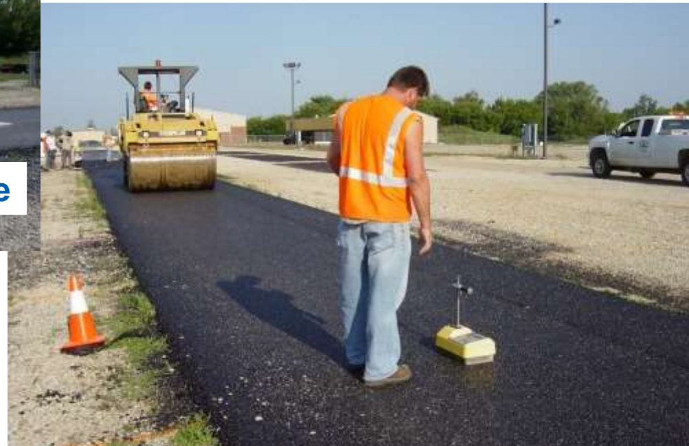
Density check with nuclear density gauge
