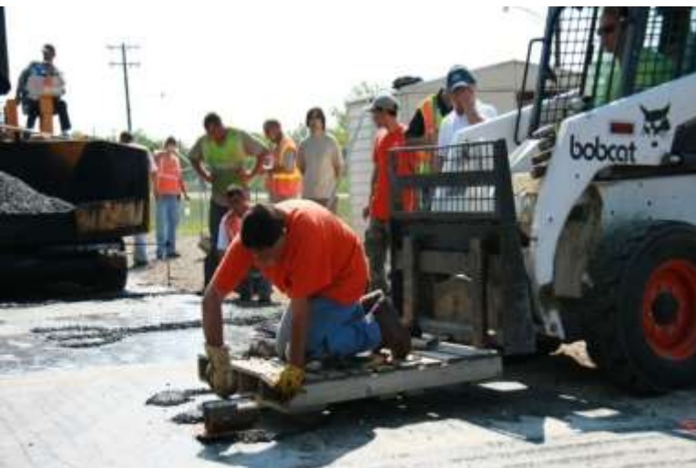
Strain gauge installation
