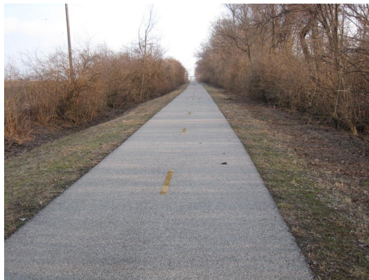
Figure D.38. Good edge support and vegetation clearance.
