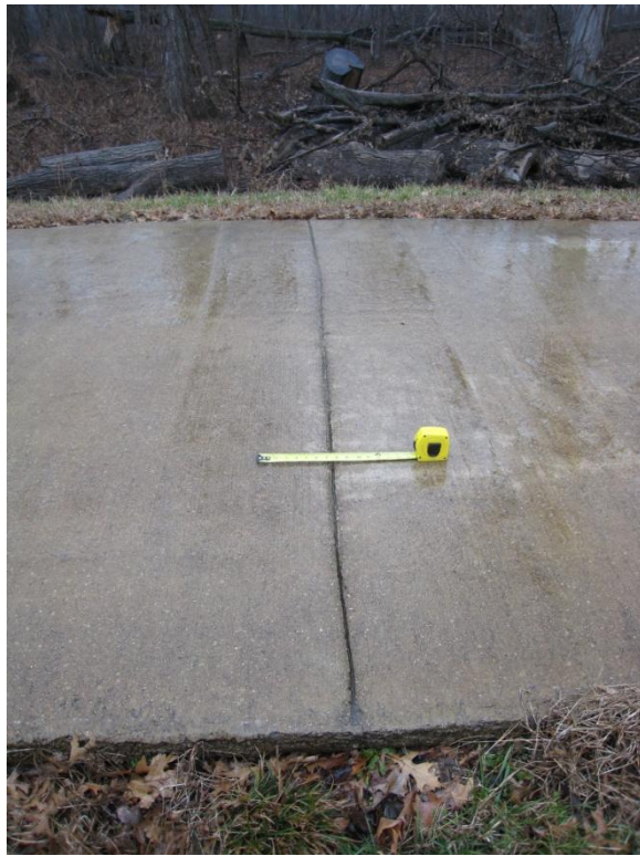
Figure D.26. Typical tooled contraction joint.
