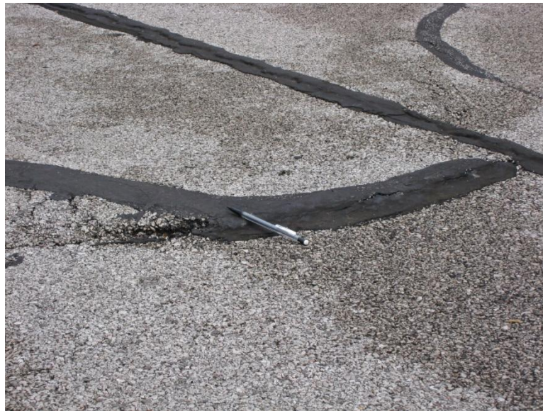
Figure D.31. Tree root infiltration.
