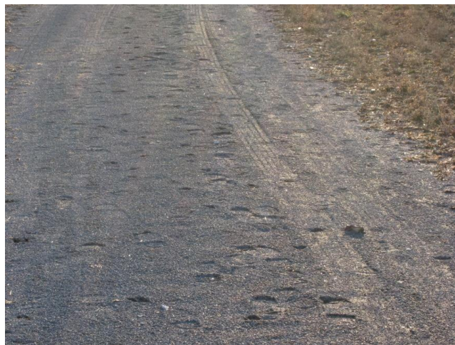
Figure D.23. Soft surface aggregate.
