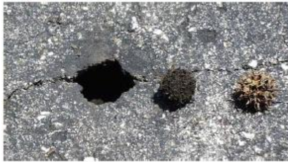
Figure 8. Pop-out caused by sweetgum ball within the HMA layer (Luttrell et al. 2004).
