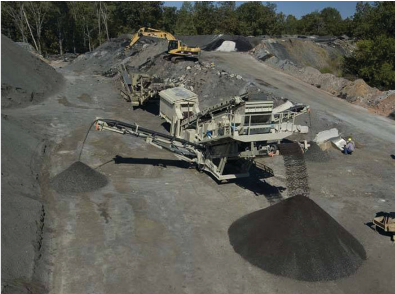
Figure 2-3. Excavator feeding material into a RAP crushing and screening process.
