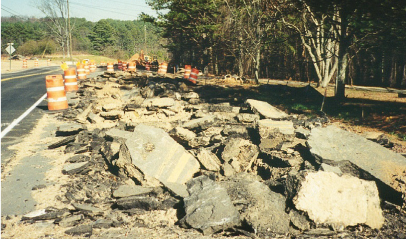
Figure 1-5. Pavement rubble from full-depth demolition of a roadway.
