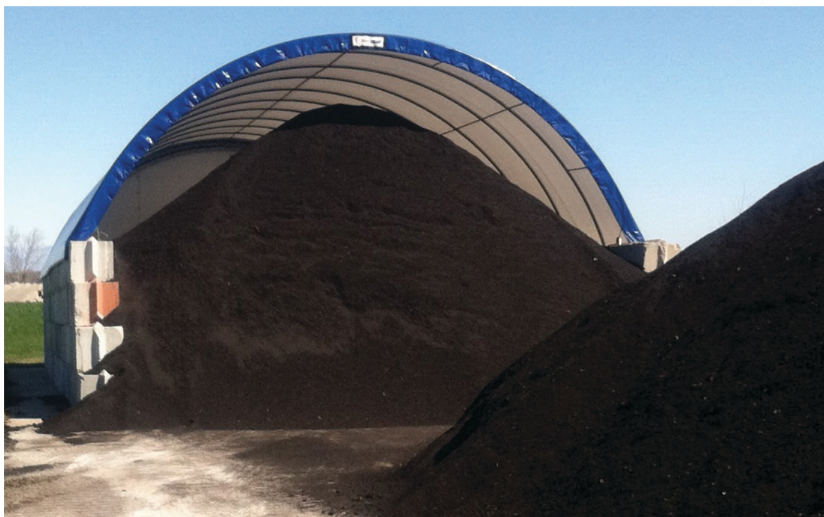
Figure 5-2. Covered RAS stockpile.
