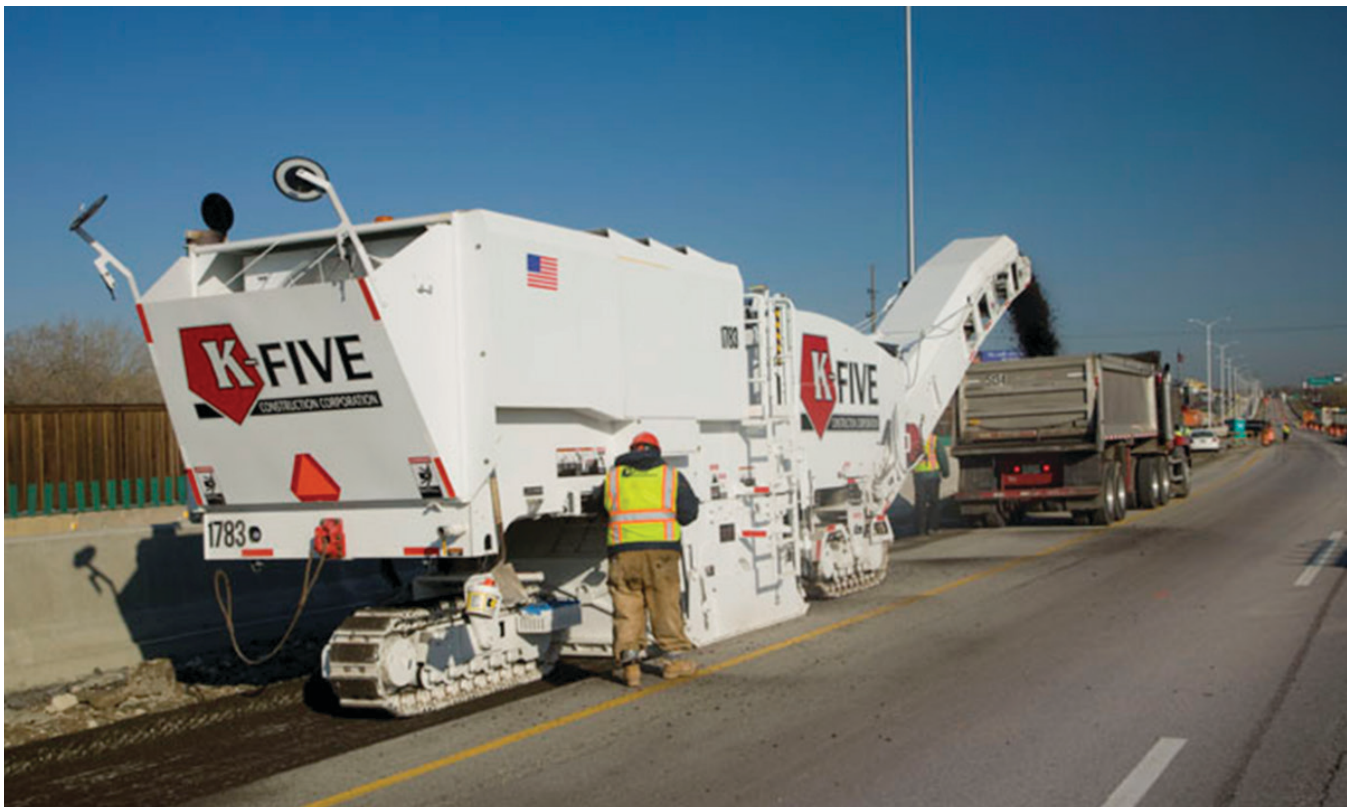
Figure 1-1. Milling machine removes asphalt pavement layers as part of pavement rehabilitation.
