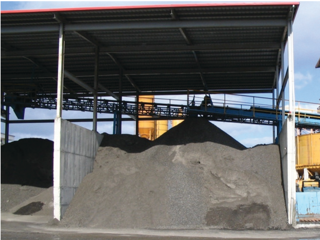
Figure 2-8. Covered stockpile to minimize moisture in RAP.
