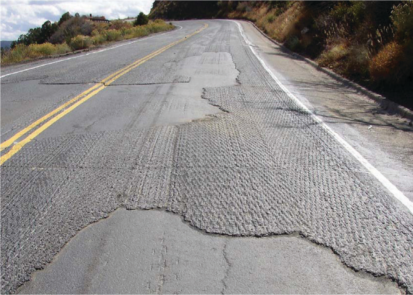
Figure 1-3. Milled pavement surface with thin scab layer that will likely lead to premature failure of the overlay. (Photo courtesy of Jim Scherocman)
