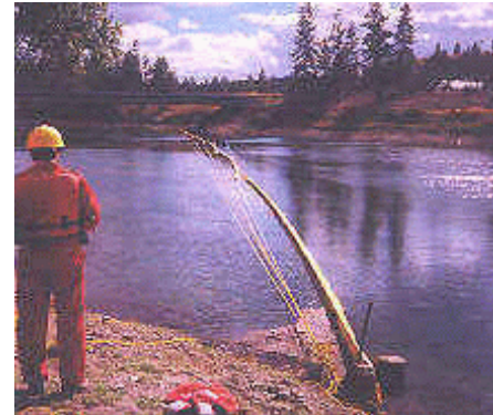
Figure 3-2: Boom deployed across Big Bear Creek.
