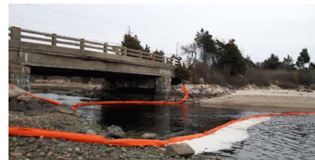
Figure 3-3: Boom deployed at Route 54 bridge crossing.
