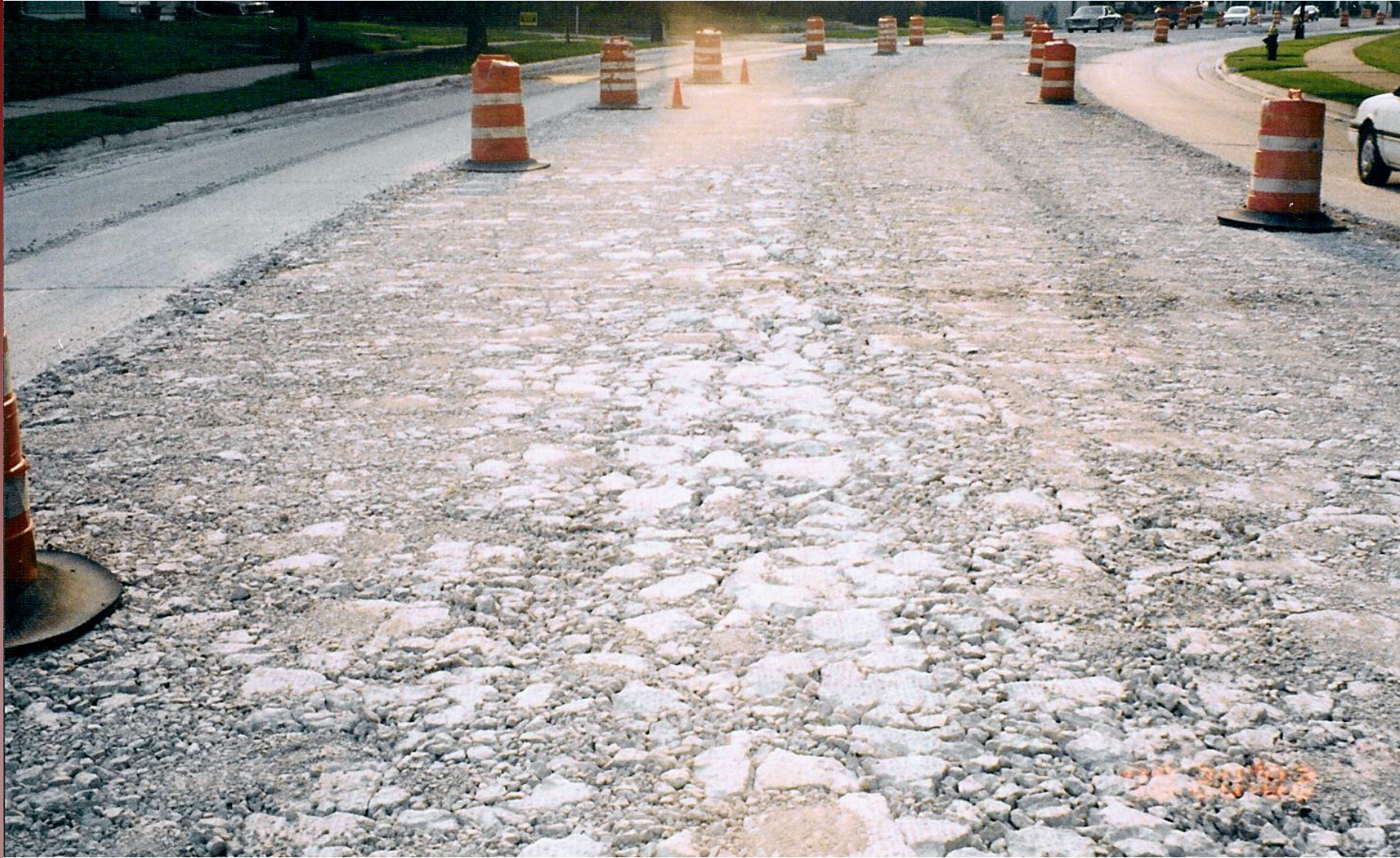
Rubblizing over a weak subgrade
