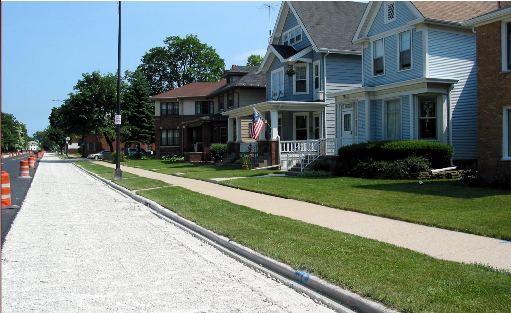
Rubblizing near homes & other buildings
