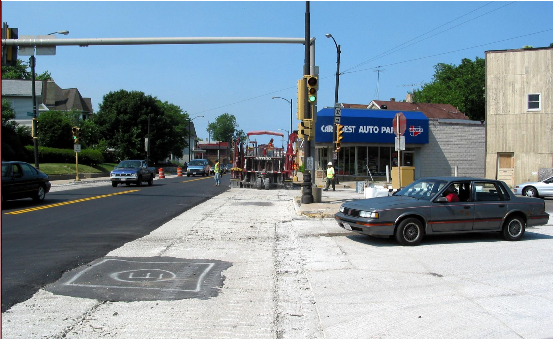
Rubblizing over and near utilities
